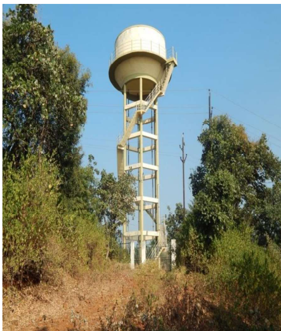
Fig-9: Overhead tank
