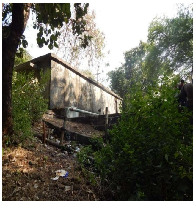
Fig-10: Water box and supply system
