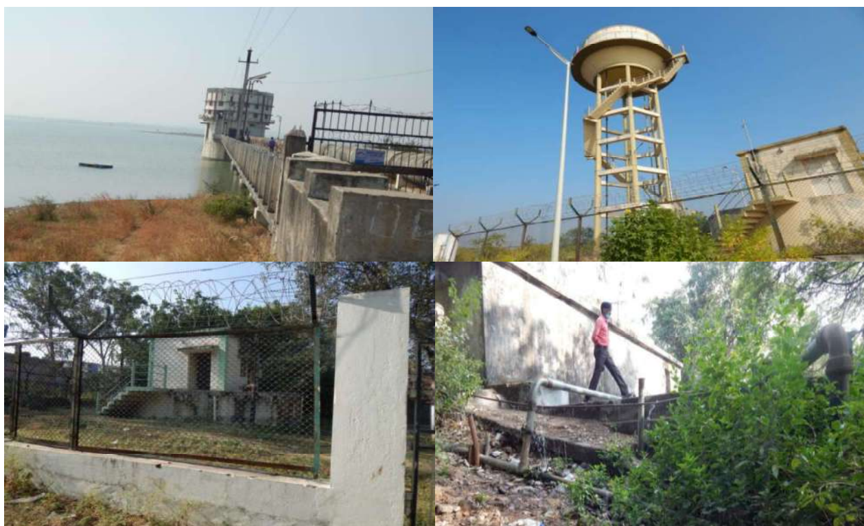
Figure-G6: Source of water and distribution system in the university.
