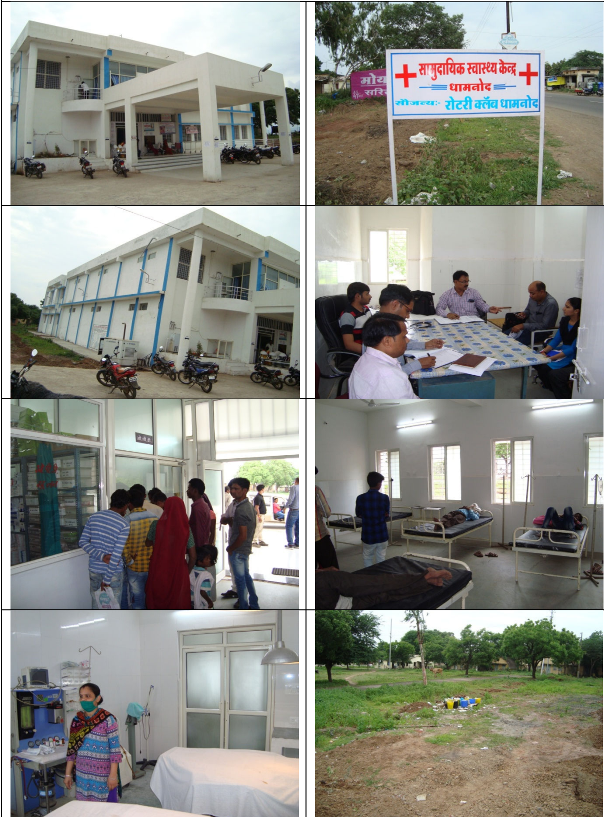
Community Health Centre (CHC) Dhamnod, District Dhar visited on 10 August, 2018
