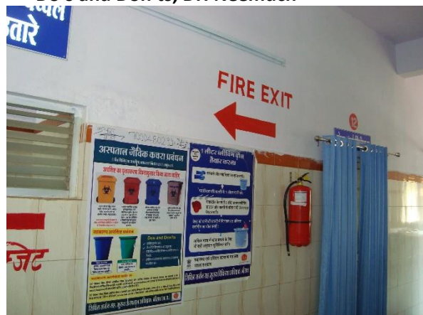
Fire Exit Instructions
