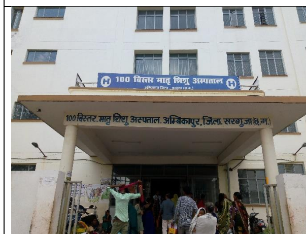
100 bedded MCH building
