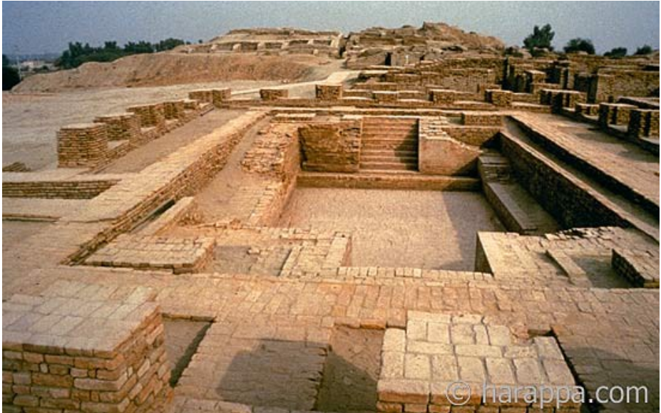
Figure 4. The “Great Bath of Mohenjo-daro.” This is the earliest public water tank in the ancient world. The tank itself measures approximately 12 meters long and 7 meters wide, with a maximum depth of 2.4 meters with two wide staircases lead down into the tank. The tank is water tight due to finely fitted bricks laid on edge with gypsum plaster. (Source: www.harappan/indus2/time.html ; obtained copyright permission from Harrappa.com))
